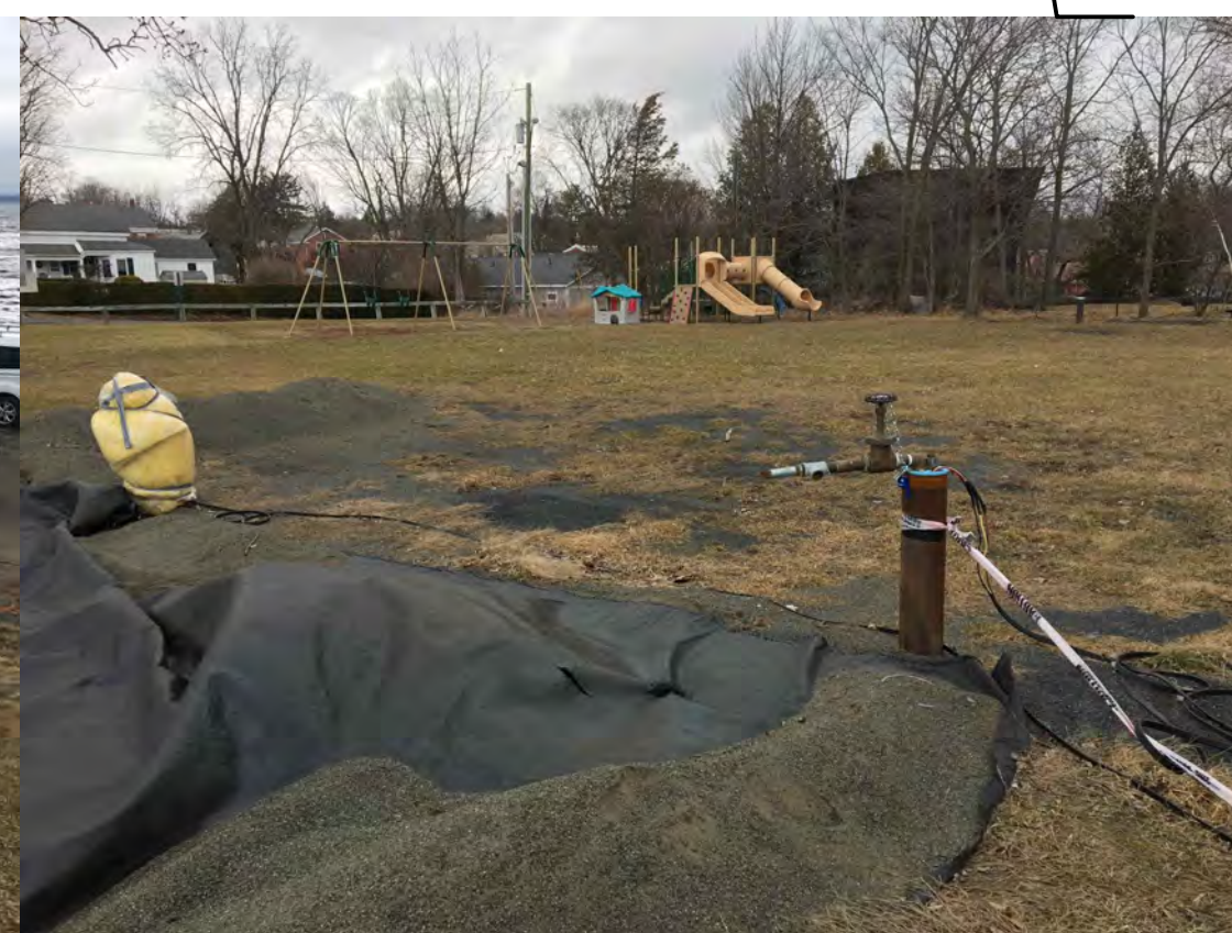
5 EXISTING WELL #1 AND #3 C-2 DATE: MARCH 1st 2017
