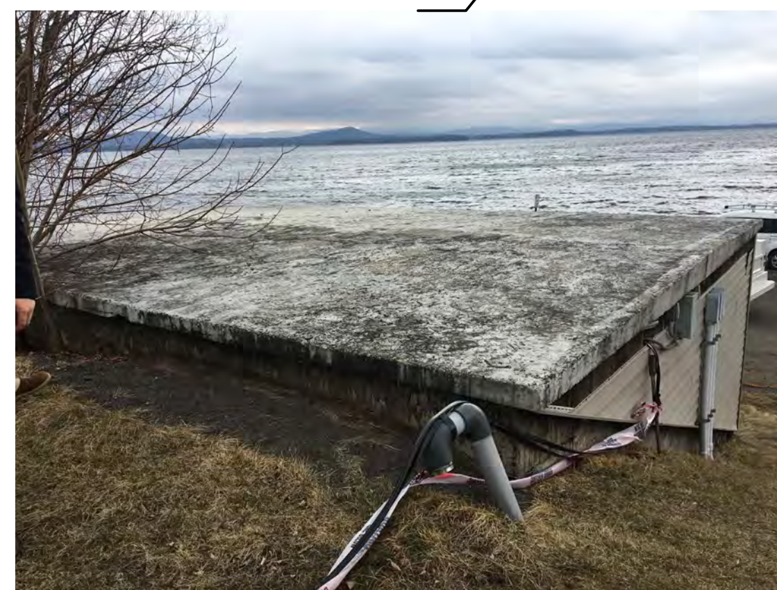
3 EXISTING ROOF PLATFORM C-2 DATE: MARCH 1st 2017
